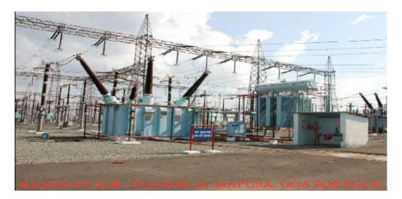
The Project involves construction of 5 nos. of 400 KV Bays including Line & AT under breaker and half scheme and 8 nos. of 220 KV Bays under Double Mains & Transfer bus scheme. The Sub-stations was SCADA controlled.
