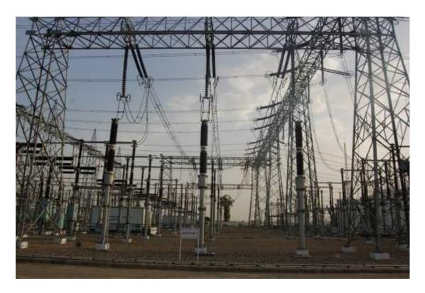
The Project involves construction of 5 nos. of 400 KV Bays including Line & AT under breaker and half scheme and 8 nos. of 220 KV Bays under Double Mains & Transfer bus scheme. The Sub-stations was SCADA controlled. Under extreme site conditions and facing multiple challenges, the work was carried out by a team of professionals with the highest International Standard.
